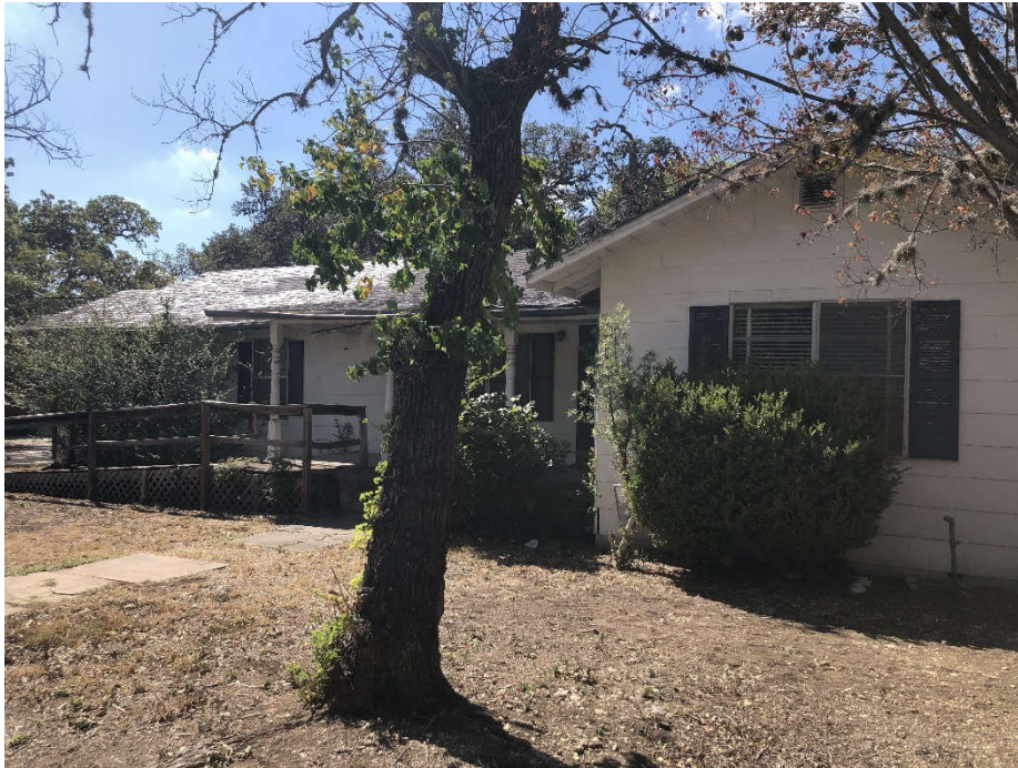
PHOTO 1: Shows the former residence located at 245 Live Oak Street in Boerne, Texas.
