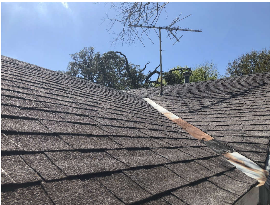
PHOTO 10: Shows the composite, shingle roof system (Samples 28-30). Testing of this material did not indicate the presence of asbestos.
